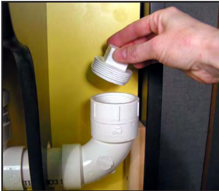
*Checking the Clean-Out for Clogs*
