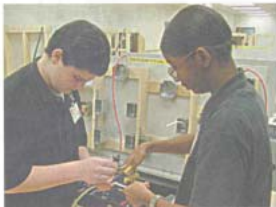
Students Ray Sittner and Shari Oden, both 17 years old, learn to wire a house for electricity at the Construction Careers Center in St. Louis.
