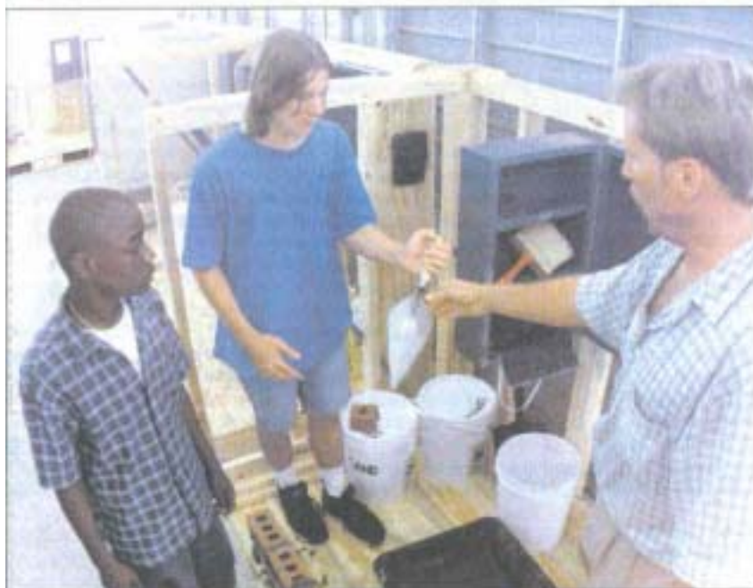
Luckson Regest, left, and John Hurhula take a few last-minute directions on mixing cement from instructor Edward Klimowich at Key West High School's construction-trades lab Tuesday.
